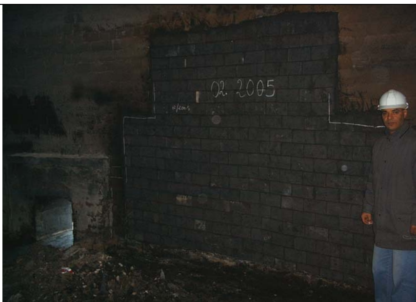
Maintenance work at a concrete Reactor wall
