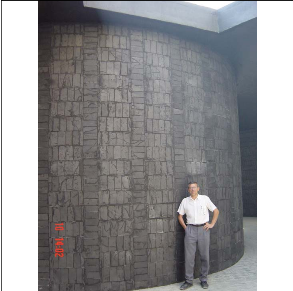
Inner Ring wall of SIAPE-Reactor
