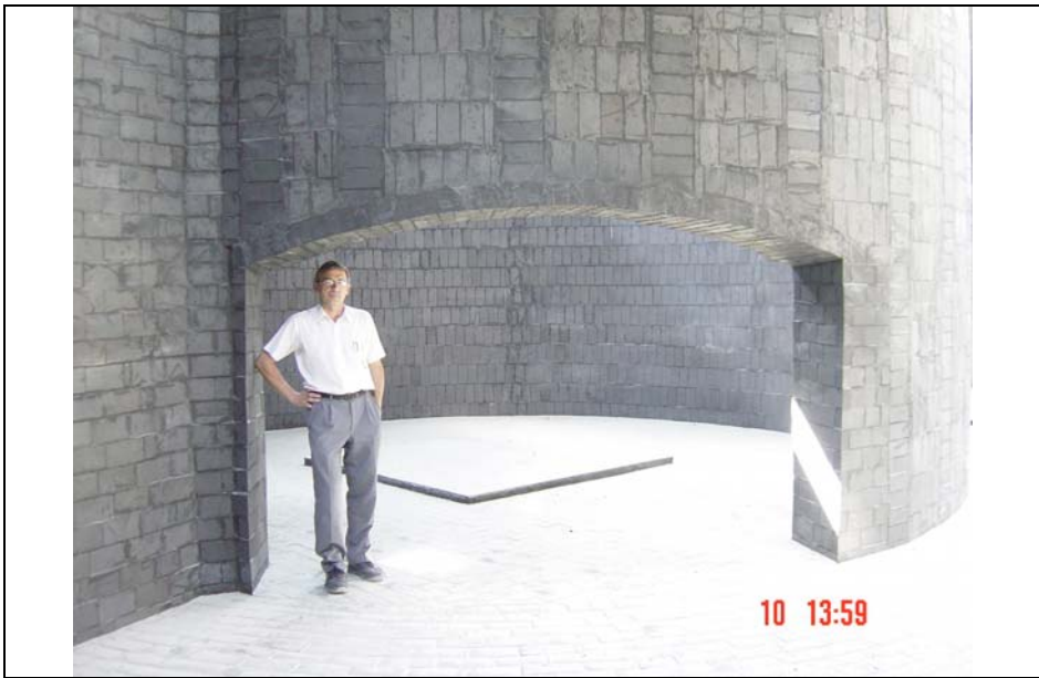
Underflow in SIAPE-Reactor
