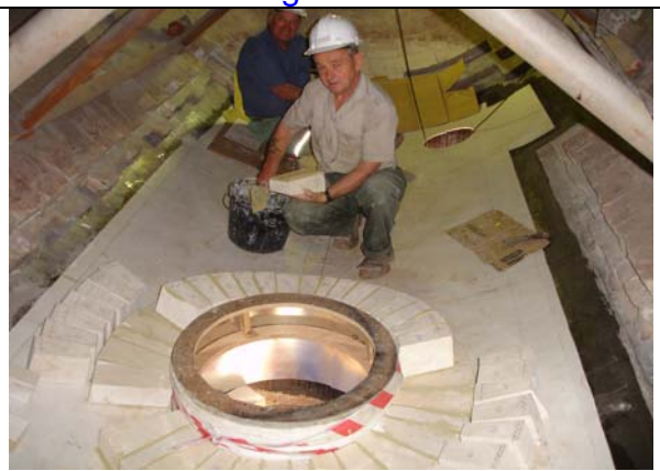
Partial Relining of Autoclave
