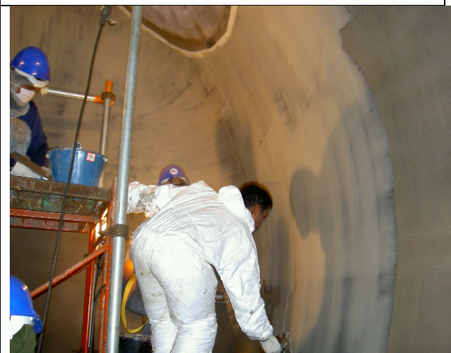
Troweled on coatings
