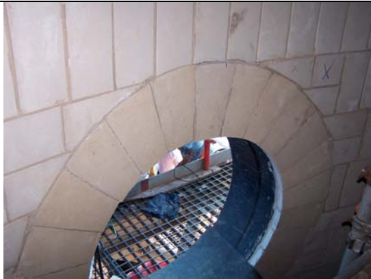
Brick lining in Flash Tanks
