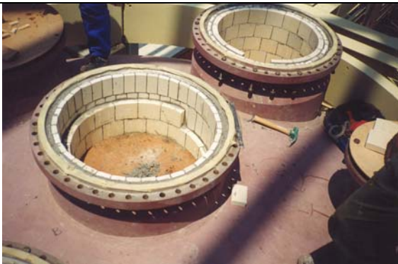
Nozzle Lining in vertical Clave
