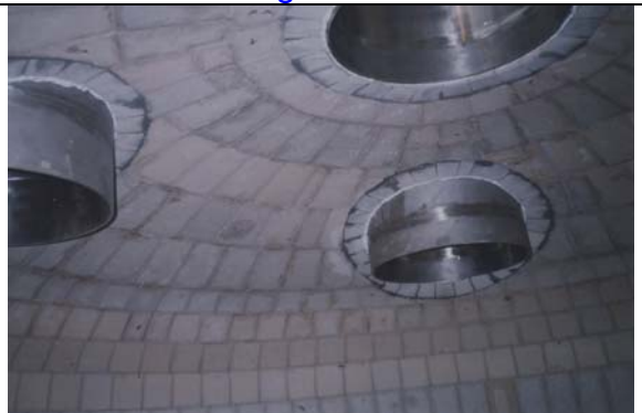
Dome Lining in vertical Clave
