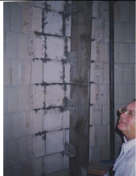
AE Mortar for bedding Baffle brackets
