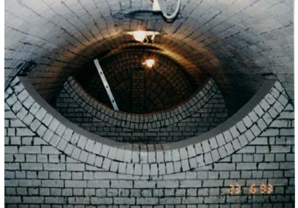
Brick-wall with inverted arch overflow
